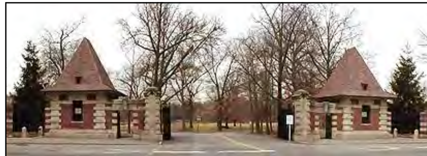
Present-day view of Ballantine Gateway, looking west across Lake Street.
