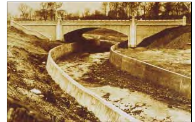
Second River channel during construction, no date. Source: Newark Public Library.
