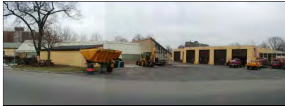
Existing maintenance facility, as seen from Brookside Drive at Heller Parkway.
