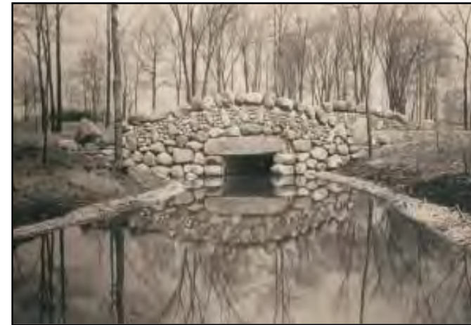
Figure 8-3: “Cobble Bridge,” between Ballantine Gates and Abington Pool. JCO photograph, 30 May 1901. Source: Photograph #2121-73,
