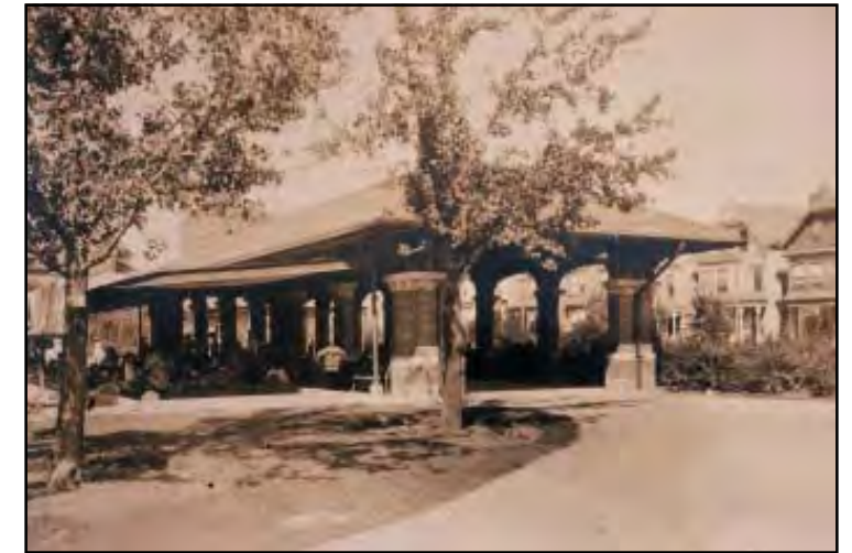
Figure 4-3: Sand-Court Shelter in the Playground, Southern Division. JCO photograph, 13 August 1902. Source: Photograph #2121-128, ONHS.
