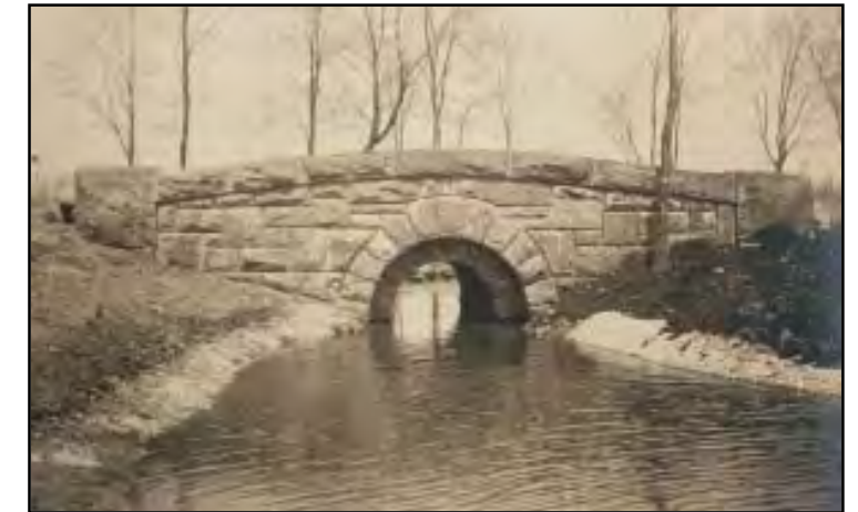
Figure 8-4: “Brownstone” footbridge near Ballantine Gates. JCO photograph, 30 May 1901. Source: Photograph # 2121-74, ONHS.
