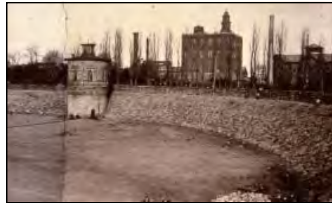
Figure 6-25: Reservoir drained, c. 1925. Source: courtesy James Lecky.
