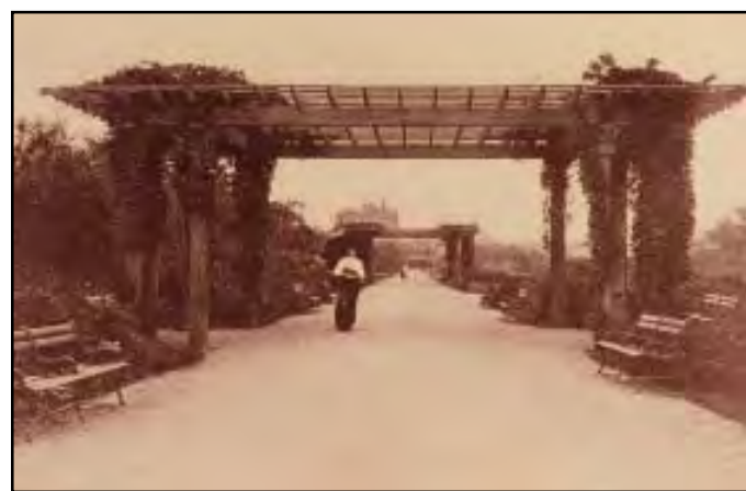
Figure 6-30: Arbors along Promenade, c. 1900. Source: Kelsey, The First County Park System , after p.232.
