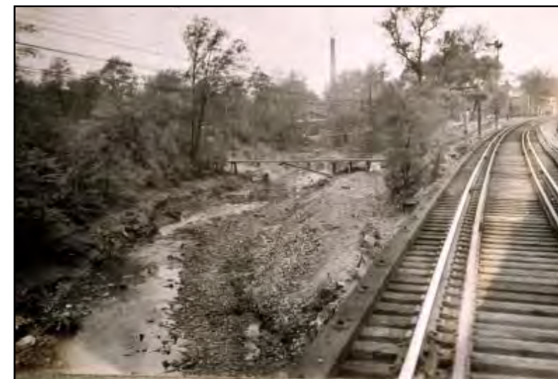
Figure 9-4: Railroad tracks near Second River. c.1925. Source: Photograph #2121-204 (second album), ONHS.
