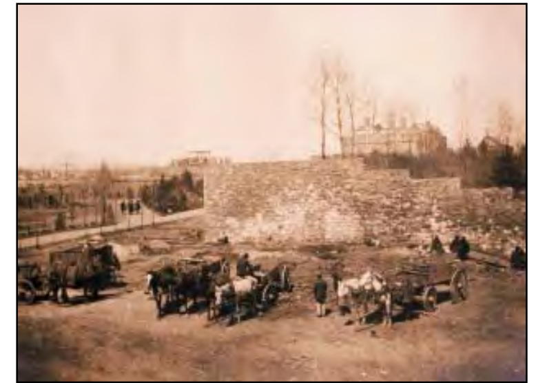
Figure 4-1: Work crew and their carts beneath High Mound wall in the Southern Division. In the background can be seen the path next to the Statuary garden. JCO photograph, 9 April 1900. Source: Photograph #2121-39, ONHS.
