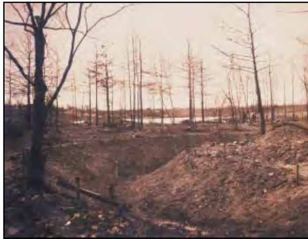
Figure 5-10: Water course in the Northern Division under construction. JCO photograph, 9 April 1900. Source: Photograph #2121-45, ONHS.
