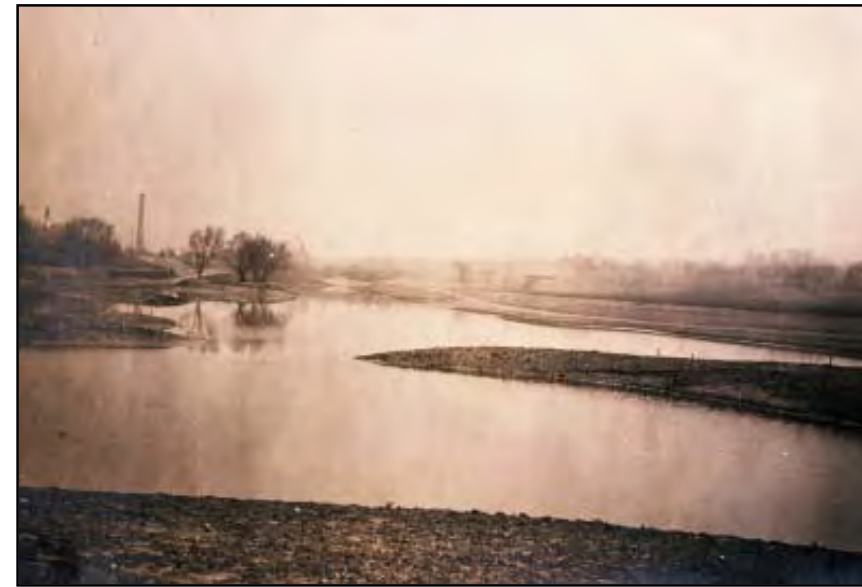
Figure 7-3: Looking north over newly constructed lake between two islands. Lake is not yet connected through to the Southern Division. Playfield is to the right. JCO photograph, 30 May 1901. Source: Photograph #2121-69, ONHS.
