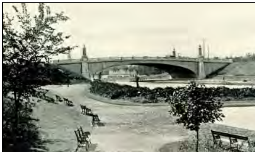
Figure 7-9: Park Avenue [Midlake] Bridge. c. 1906. Source: 1907 Annual Report , p. 12.
