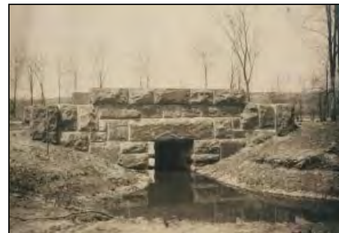
Figure 8-5: “Brownstone Lintel” footbridge near north end of brook. JCO photograph, 30 May 1901. Source: Photograph #2121-78, ONHS.
