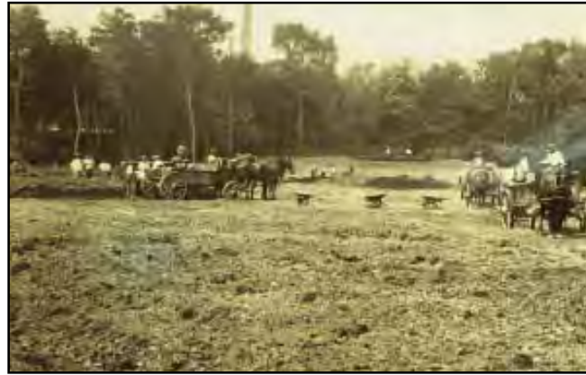
Figure 9-7: Construction of Hendricks Field, green #5, August 1927. Source: Newark Public Library photograph collection.
