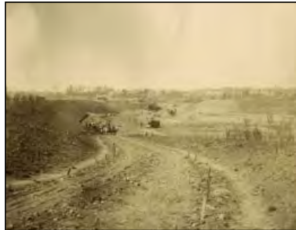
Figure 5-11: Looking south-southwest from Fourth Avenue toward the site of the Fifth Avenue underpass. Grading work along the Lake Street slope is in process. JCO photograph, 7 May 1900. Source: Photograph #2121-49.
