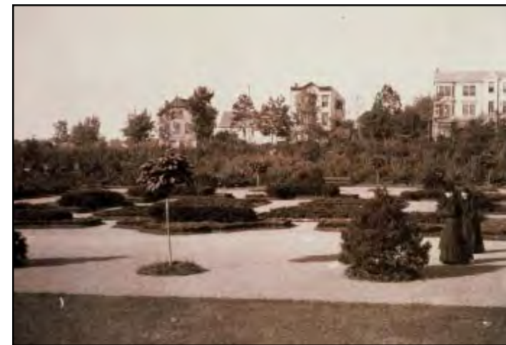
Figure 6-26: Looking north over the Box Garden. JCO photograph, 1898. Source: Photograph #2121-118, ONHS.
