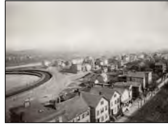
Figure 1-6: View from Clifton and Seventh Avenues, 1896. Source: 1898-99 Annual Report , after p. 10.
