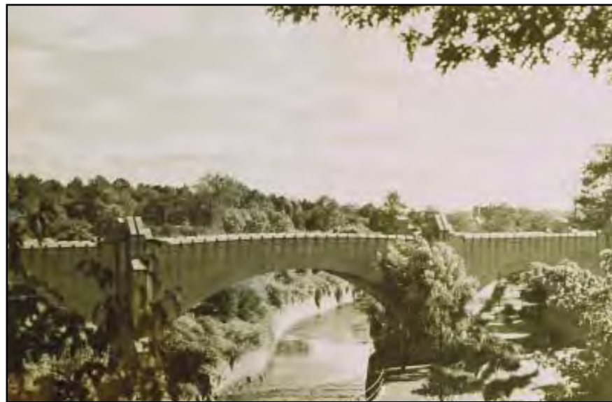
Figure 9-5: Bridge over Second River. Source Newark Public Library photograph collection.
