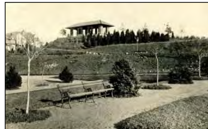
Figure 4-4: Parker Street Shelter, 1899. Source: 1898-99 Annual Report, after p. 14.
