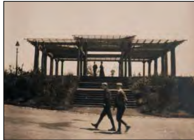
Figure 6-16: Looking east at Arbor and steps on Clifton Concourse Hill. JCO photograph, 7 May 1900. Source: Photograph #2121-55, ONHS.
