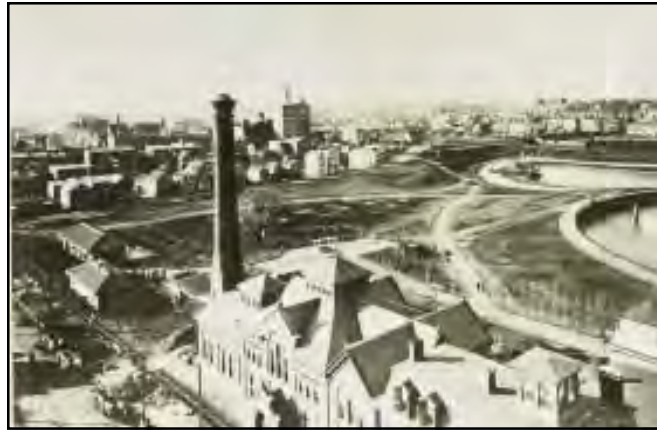
Figure 1-5: View south looking toward Eighth Avenue with the Pumping Station in the foreground and the edge of the Reservoir to the right, pre 1896. Source: Newark Public Library.
