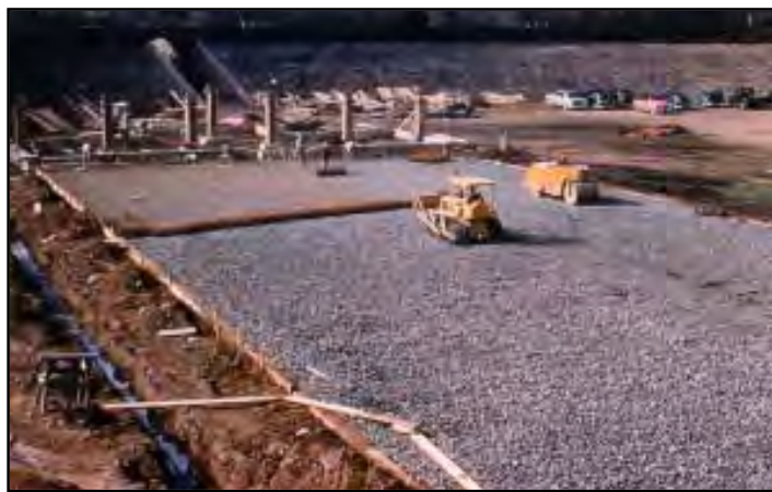
Figure 10-2: Construction of the skating rink in the former Reservoir, indicating the road cut in the embankment. c. 1955. Source: courtesy James Lecky.
