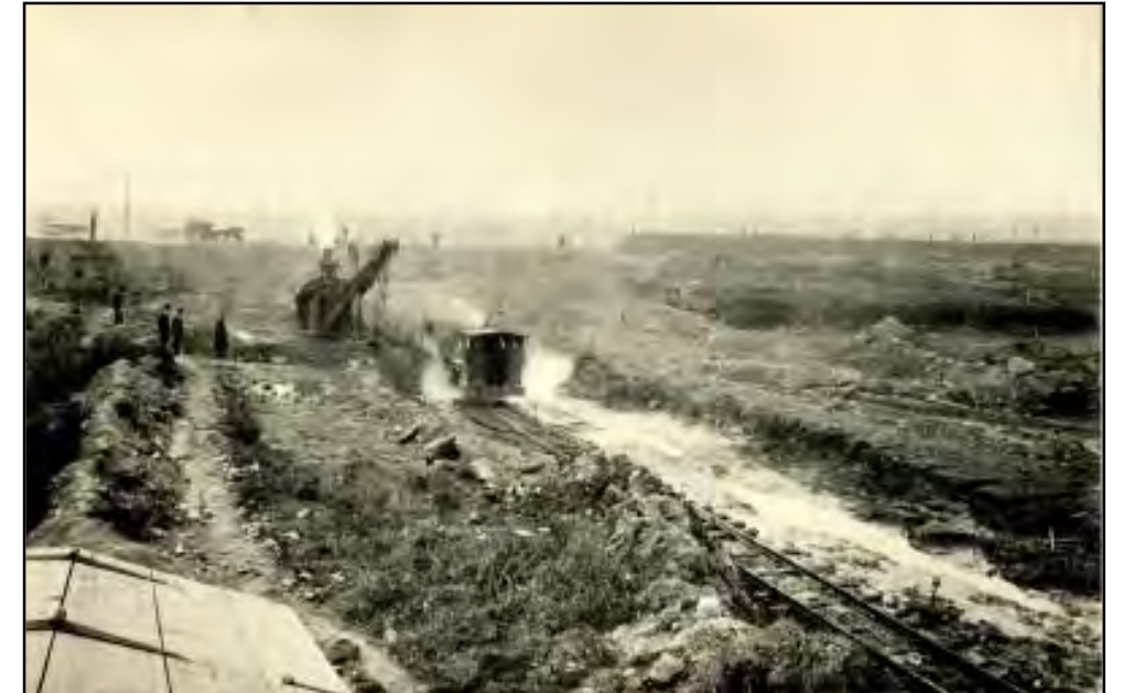
Figure 7-1: Steam shovel at work excavating the lake in the Middle Division, 1899. Source: 1898-9 Annual Report , after p. 38.
