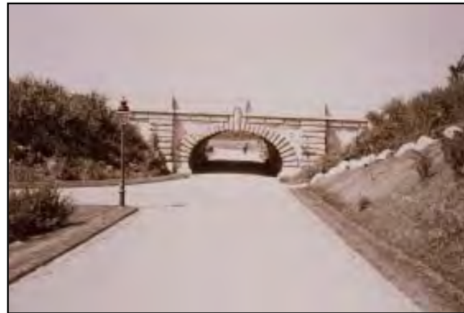
Figure 6-10: Looking west through the East Arch. E.F. Keller photograph, c.1901. Source: Photograph #2121-141, ONHS.
