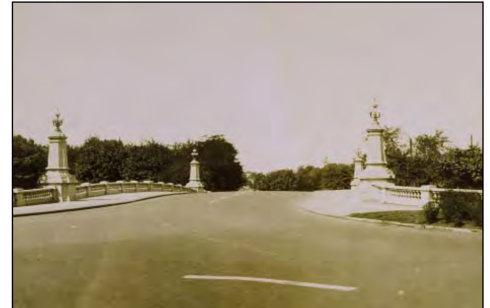
Figure 5-13: Looking west across the Park Avenue Bridge. Source: Newark Public Library photograph collection, no date.
