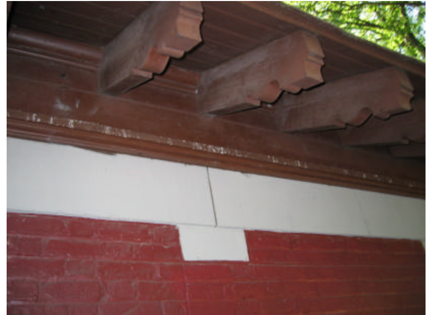
Photo 64 Wood and metal cornice on the front façade of the building.
