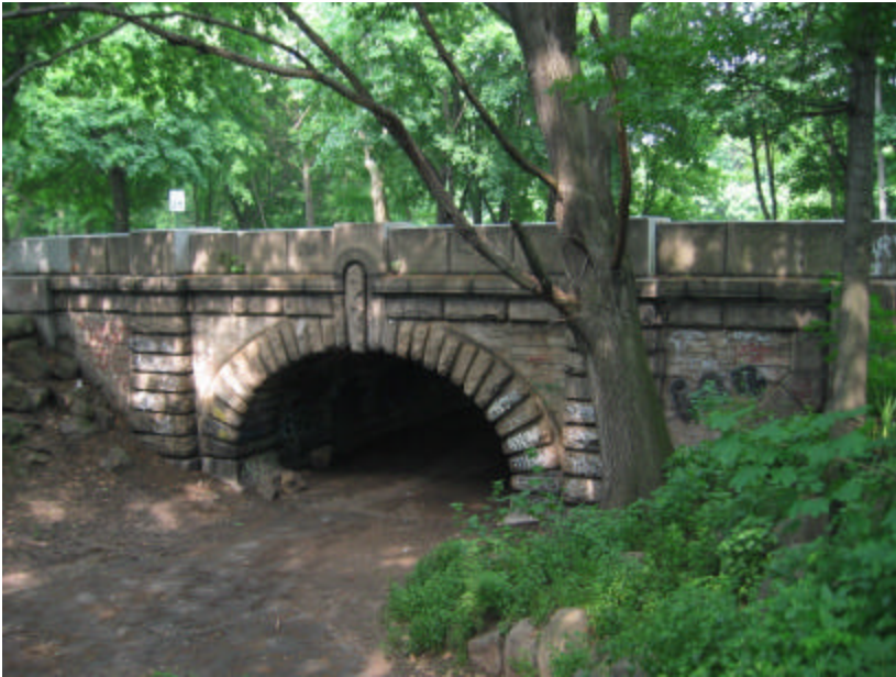
Photo 32 The east side of Subway 1; note the different stonework, a quarry-faced finish on this side of the underpass.
