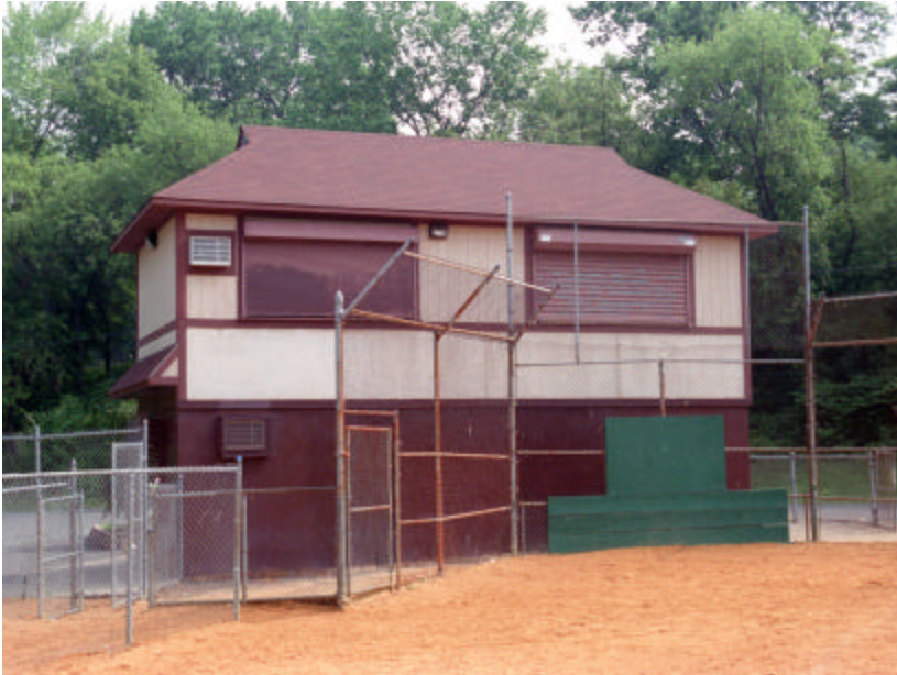
Photo 138 Overall view of the Rick Cerone field house with the press box on the second floor; note that the building is in good condition.
