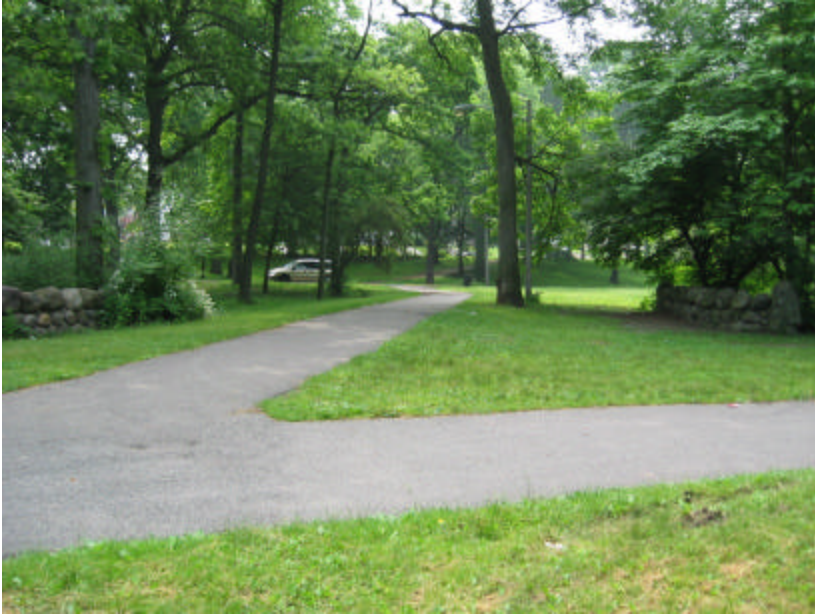
Photo 170 The Crossover Drive Bridge; note the width of bridge.
