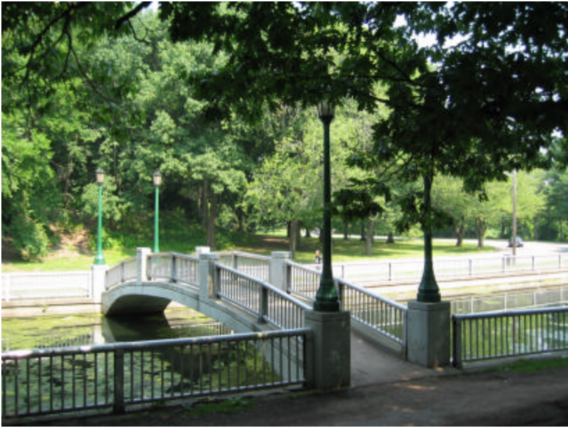
Photo 83 The concrete arched footbridge crossing over the channel between the two sections of Branch Brook Lake; note the aluminum railing and lamp posts.
