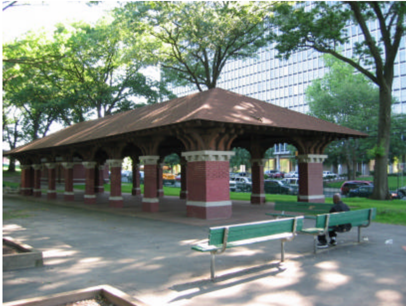
Photo 13 View of the shelter looking northeast; note that it is accessible from all sides.
