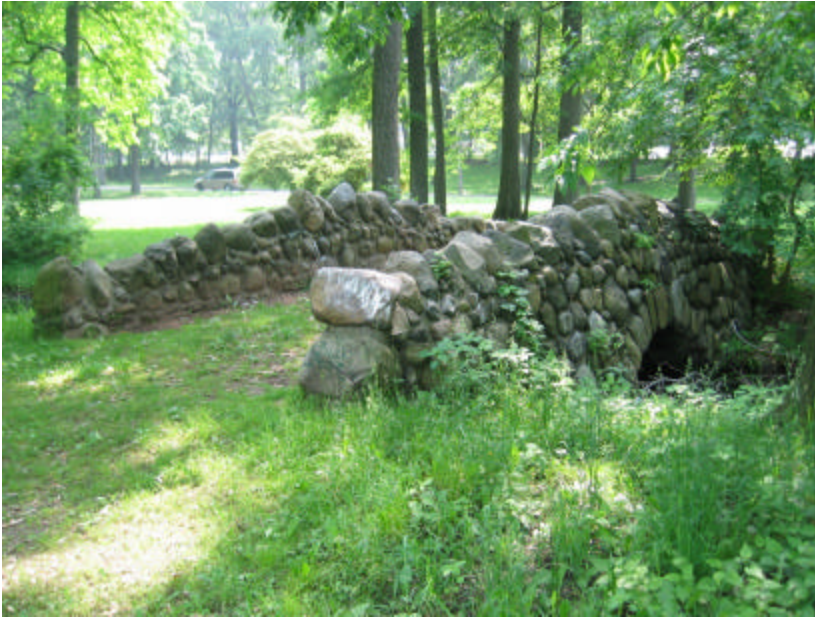
Photo 160 The Laurel Wood Boulder Bridge; note the overgrowth of vegetation around the site.
