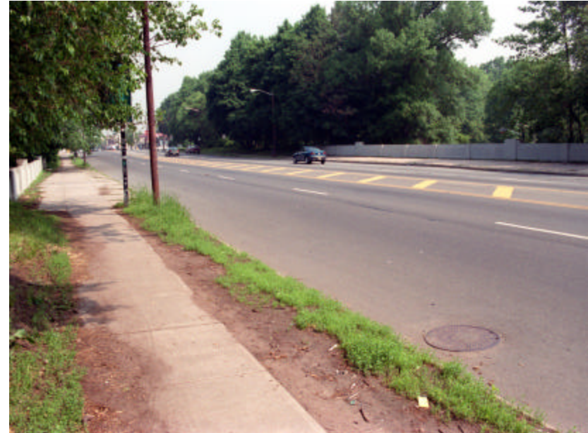
Photo 142 Bloomfield Avenue over the top of the bridge; note the erosion along the sidewalks just east of the bridge.
