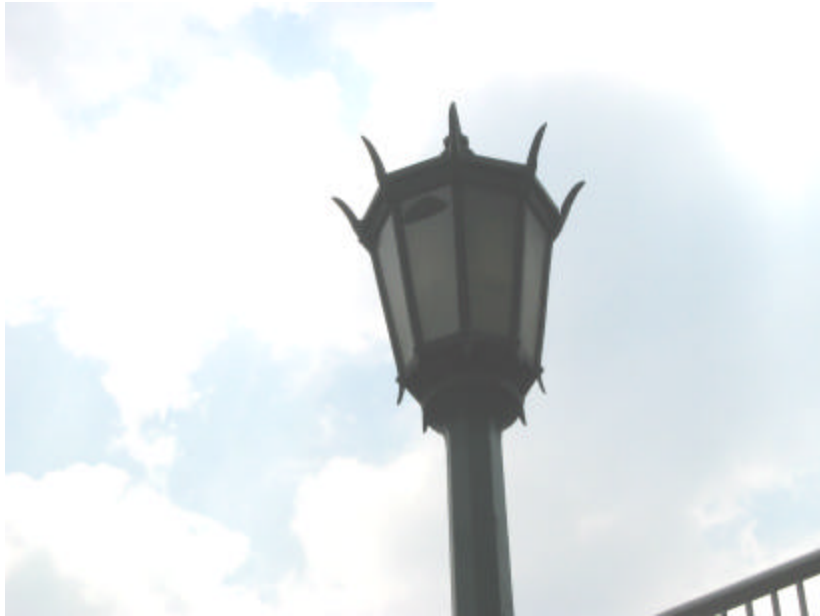
Photo 87 A section of broken glass in the lamppost on the southwest side of the footbridge.
