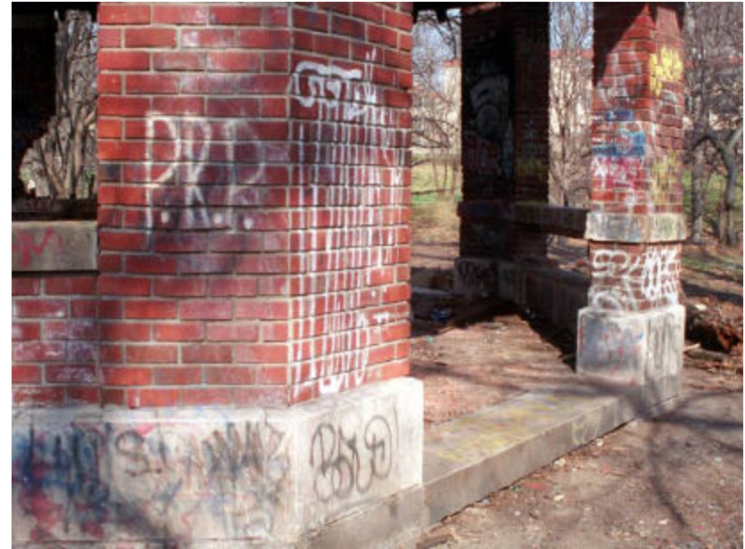
Photo 113 Detail of The Octagon Shelter, column No. 5.5, showing reconstructed brick column.
