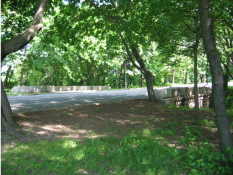
Photo 26 The paved asphalt roadway over subway.
