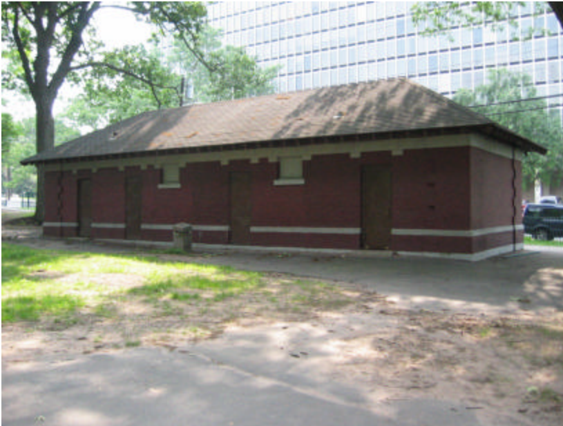
Photo 57 The front façade of the comfort station.
