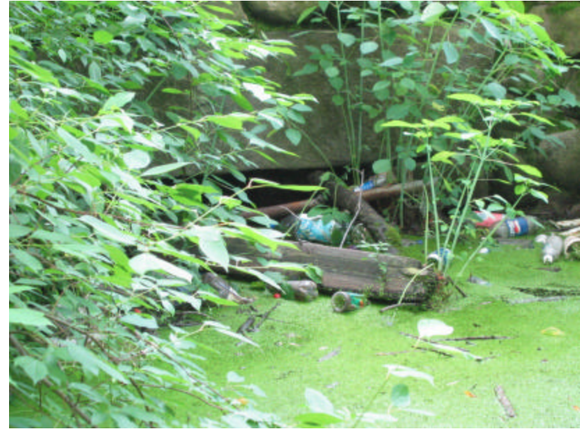
Photo 173 Organic debris and garbage clogging the culvert on the north side of the bridge.
