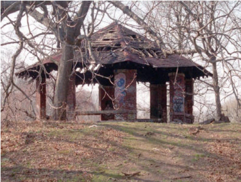
Photo 102 View of The Octagon Shelter from the south; note extensive roof damage and graffiti.
