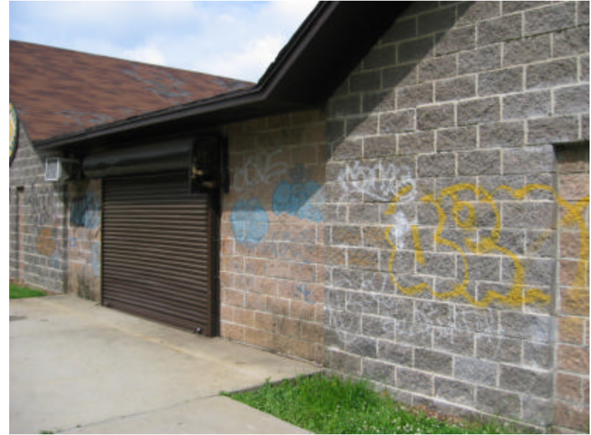
Photo 137 The east façade of the seniors' center is covered with graffiti; note the rolling steel security gates that cover the doors and windows at night.
