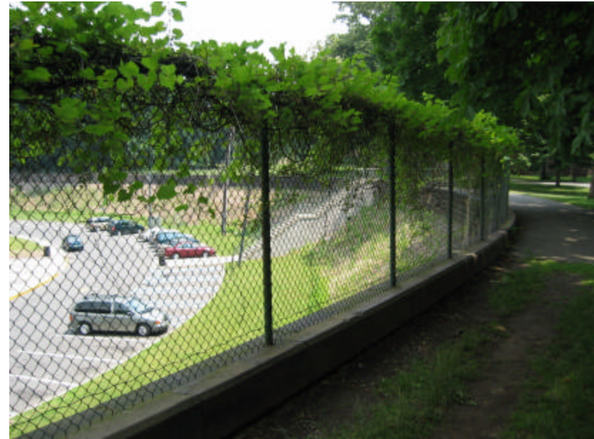
Photo 5 The wall and chain link fence surrounding the reservoir; note the vines covering the top of the fence as well as the staircase ascending from the parking lot.
