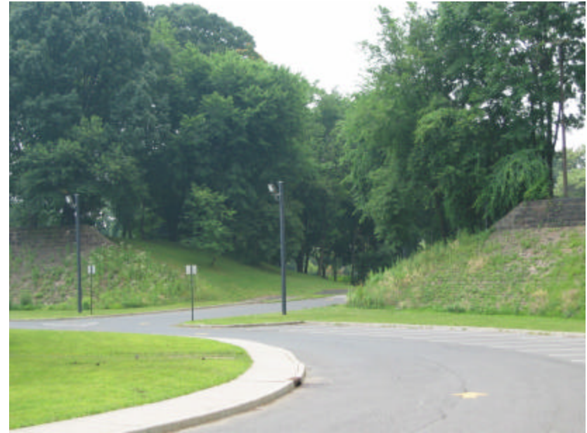
Photo 7 A cut was made in the wall so that a road and parking lot could be built.
