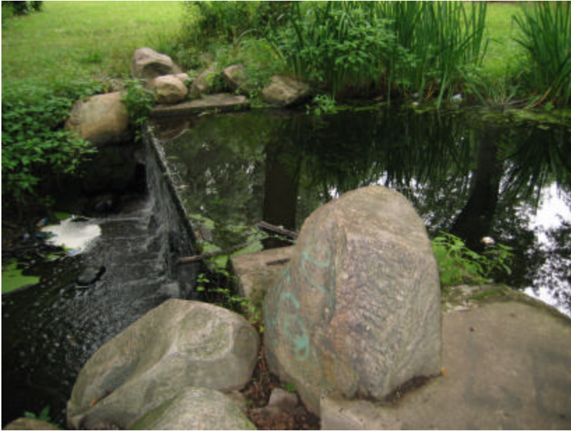
Photo 159 View of the extant concrete and fieldstone sidewalls at Weir 1 which (with the later concrete grid stabilization) continue to function along the embankments.
