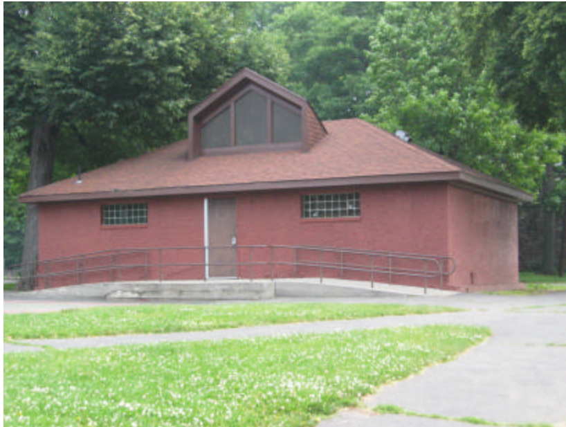
Photo 23 Overall view of the main façade of the field house; note the large skylight and glass block windows.
